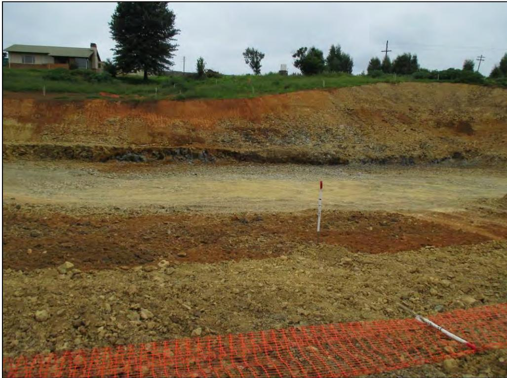
Figure 2: Excavation of pumpstation platform.
